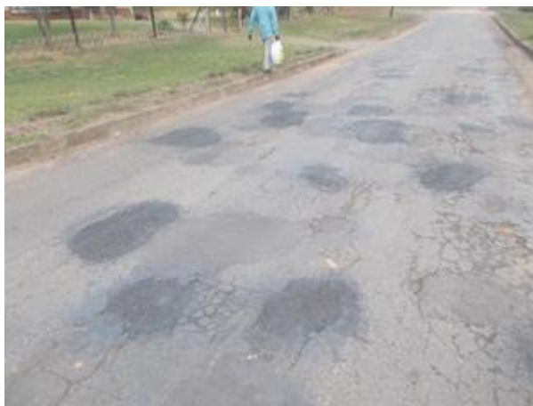
Repaired Potholes
