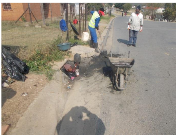
Opening & Cleaning of Drain
