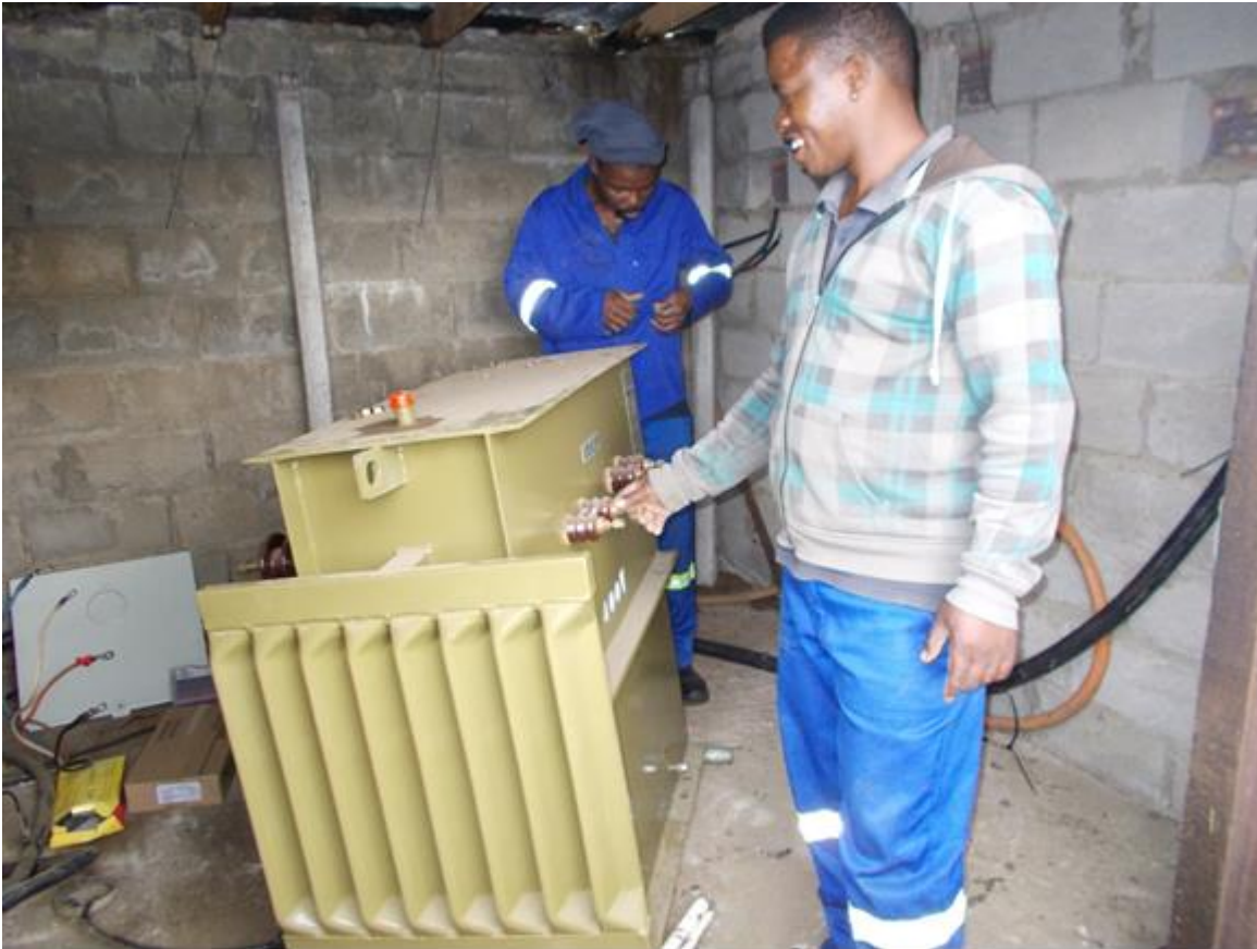
Installation of new transformer at sub N
